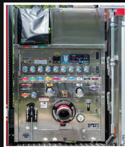
Side-Mount Pump Module (Hale)
